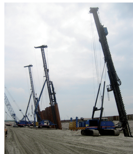
Fig. 1: A quay wall under construction at Maasvlakte 2
