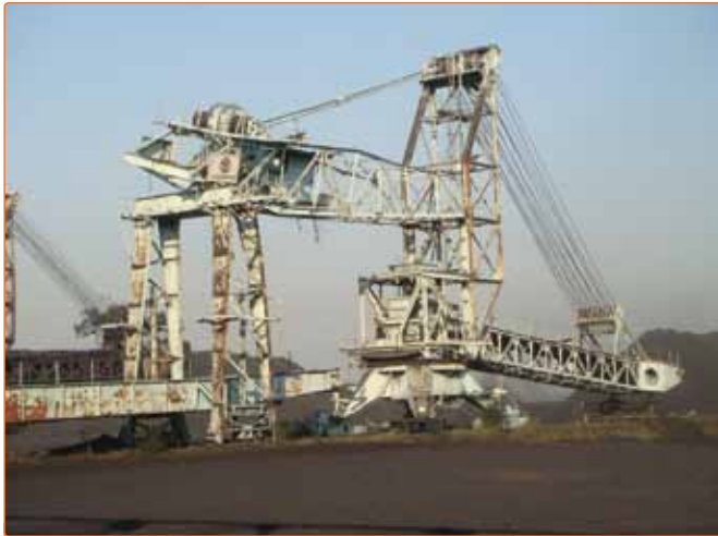
Figure 5. Before: A tired and collapsed combination bucket wheel stacker-reclaimer from 1964.
