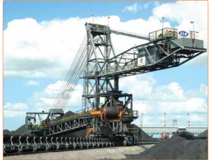
Figure 6. After: The rebuild of the SR02 machine is complete (March 2009).
