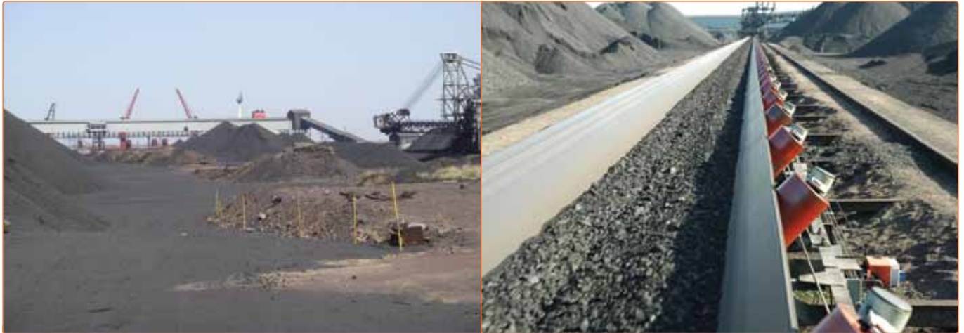
Figure 3. Conveyor C8 before and after refurbishment.
