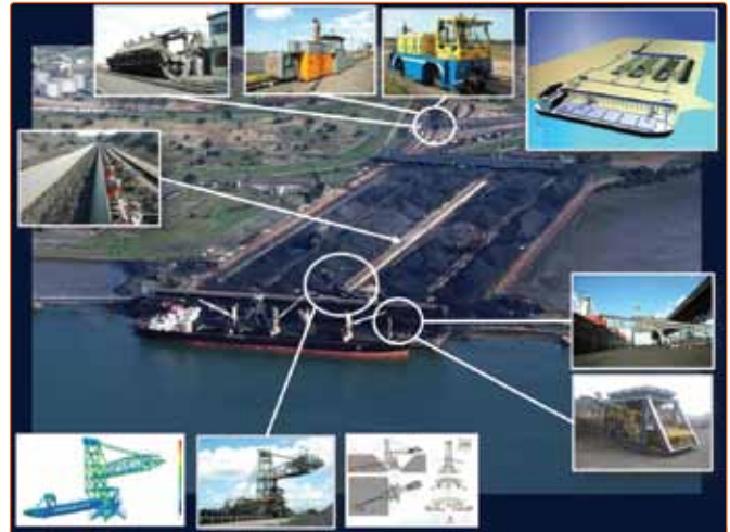
Figure 2. Photographic project overview of Phase 1 & 2.
