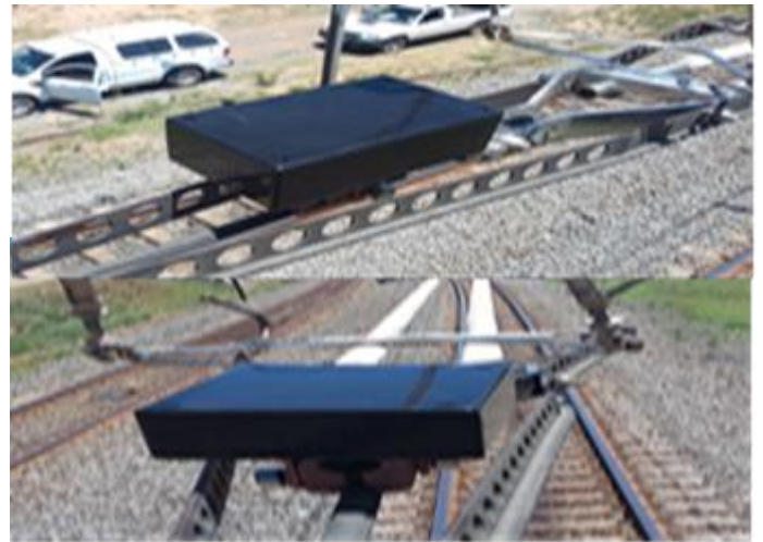
Figure 2. Accelerometer installed on the Neutral Section
