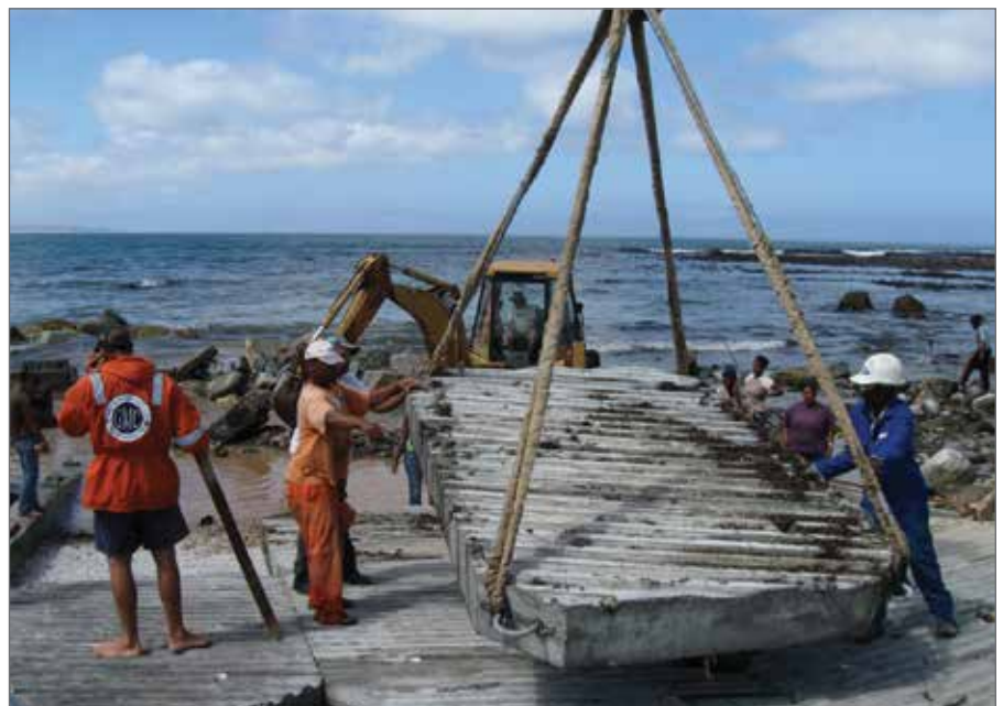
Photo 8: Placing 2 m x 3 m x 300 mm slabs at Witsands near Kommetjie
