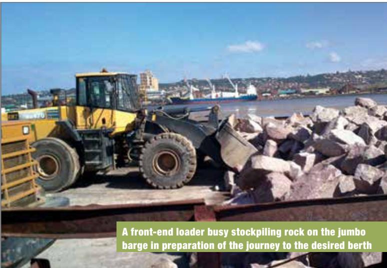
Once the barge is positioned over the dumping grid using its GPS system the front end loader places scour rock into the allocated dump blocks
