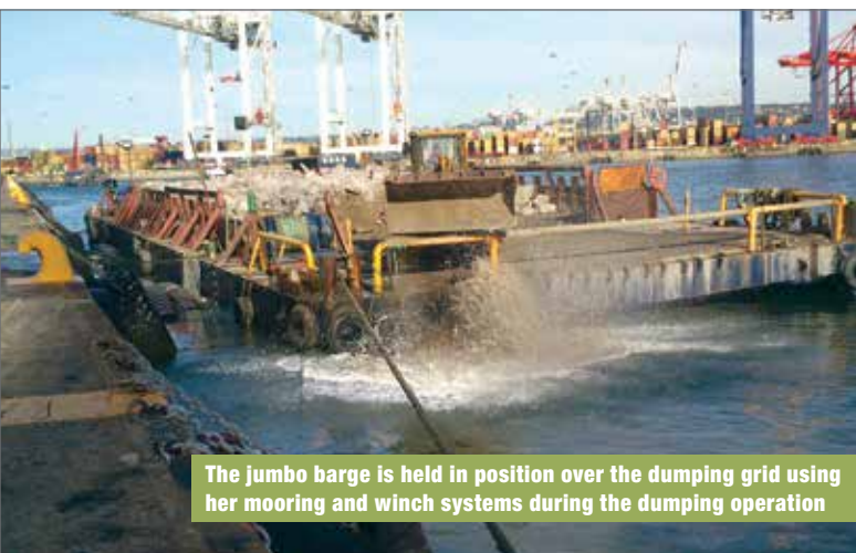
Placing the scour rocks into the desired dump blocks off the jumbo barge using a front-end loader
