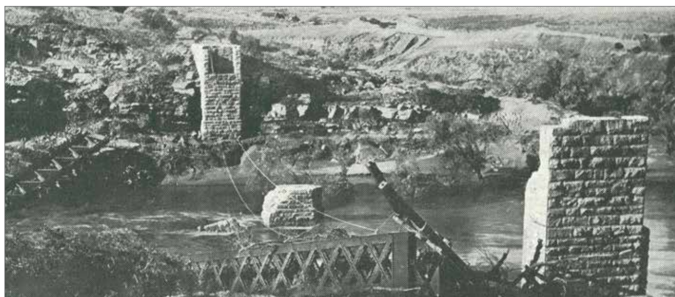
Figure 2: Kraal River Bridge (#2), shortly after being washed away on 23 March 1925, viewed from slightly downstream on the true left bank ( SA Railways and Harbours Magazine , July 1925)
