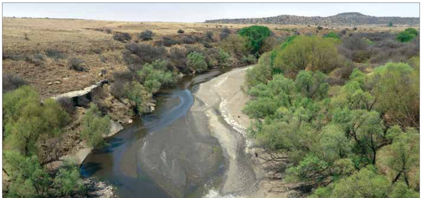
Figure 11: An upstream view from the current bridge; notice the remains of the railway bench for the temporary deviation directly to the left of the river (Photo Johannes Haarhoff 2013)
