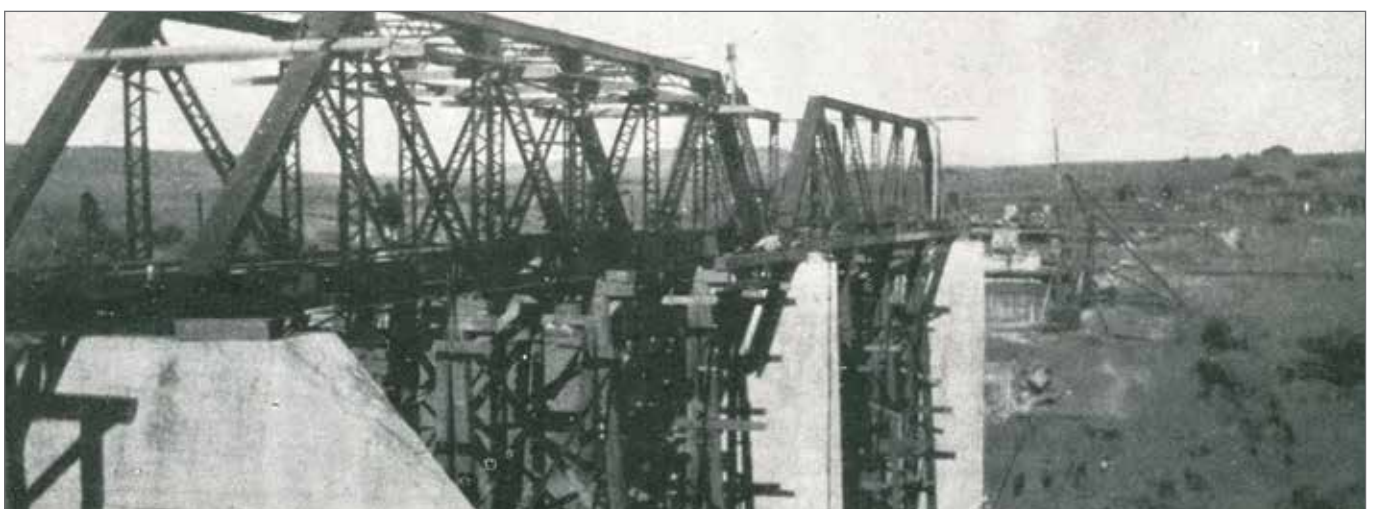
Figure 9: New permanent bridge shortly before completion, 8 June 1926; view towards Lady Grey (SA Railways and Harbours Magazine, August 1926)
