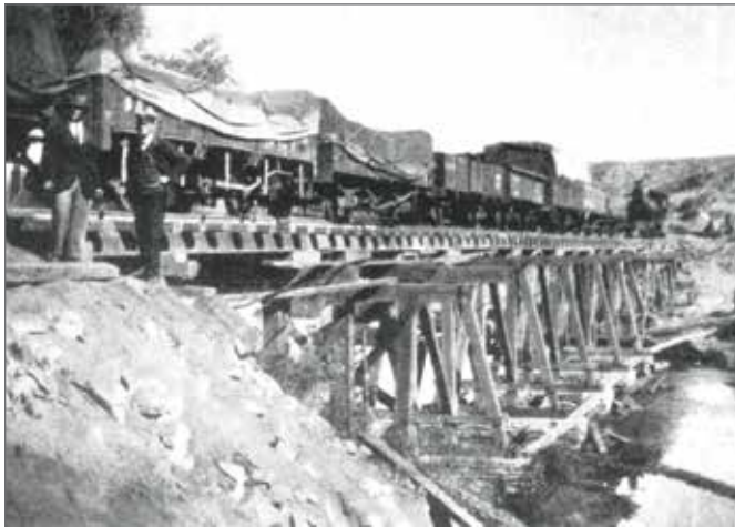
Figure 6: Temporary bridge #6, completed 25 June 1925 until washed away early March 1926 (SA Railways and Harbours Magazine, August 1926)
