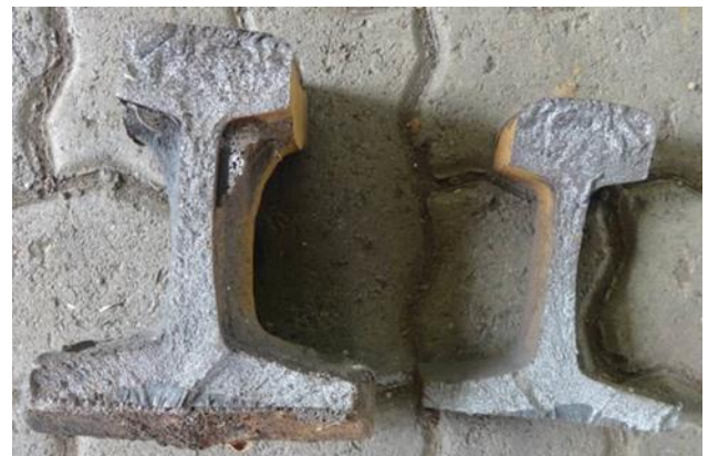
Figure 6: Typical failure on junction weld (picture taken by Lutendo Ndou TFR RTDC)
