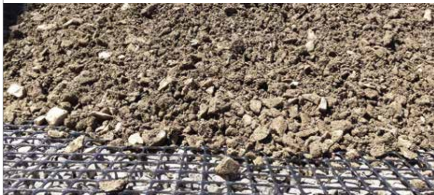
Figure 4: Construction of the geosynthetic reinforced soil raft foundation
