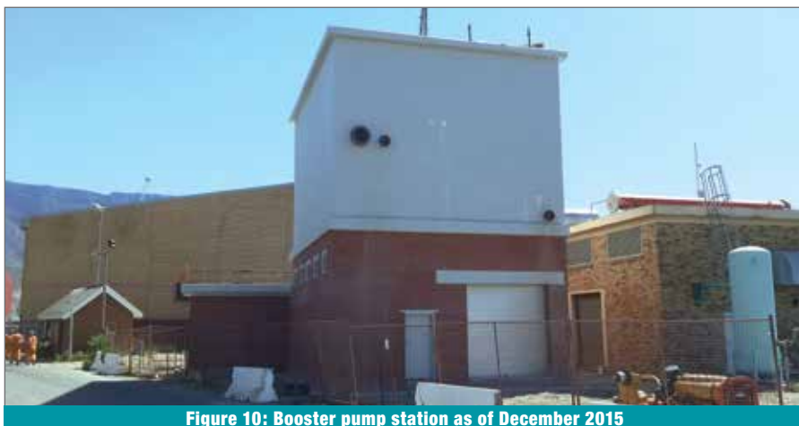
Figure 10: Booster pump station as of December 2015
