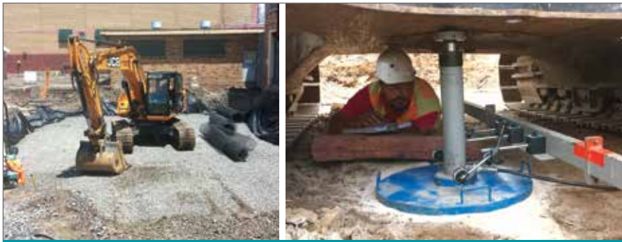
Figure 7: Plate load test undertaken during construction
