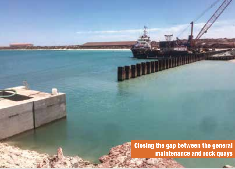
Placing of precast anchor walls
